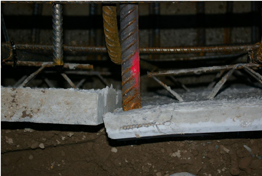
badly installed reinforcement cage
